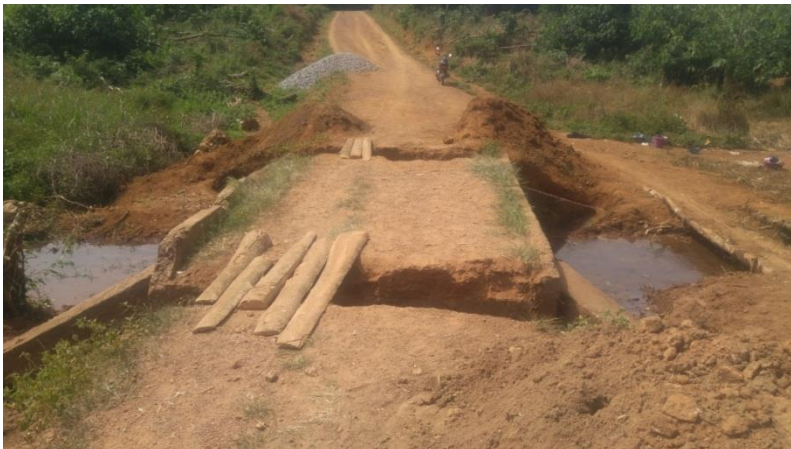
Figure 3.8: On- going Unsupervised Works to Construct Culvert
