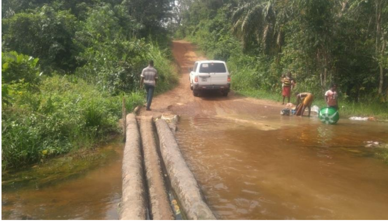
Figure 3.6: Road Becomes Impassable at Wide Stream; Steep Gradient Evident.
