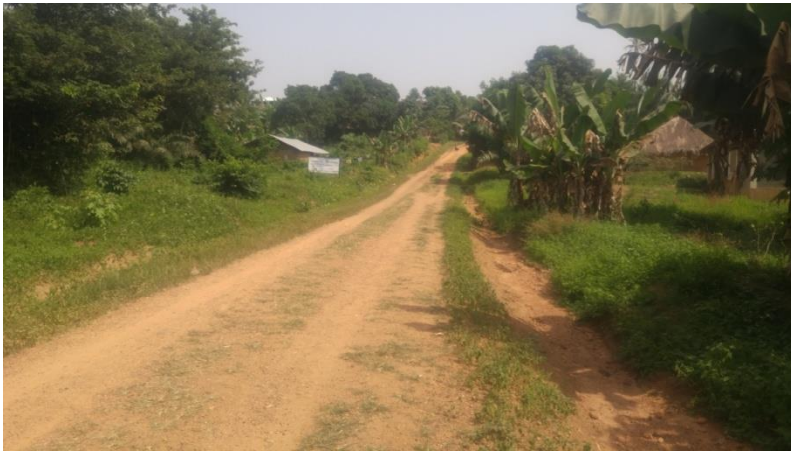
Figure 3.7: Apparent Engineered Road; Evidence of Side Drains Recently Constructed
