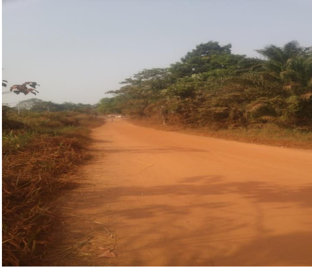
Figure 3.16: Relatively good gravel road; Overgrown Vegetation at Edge of Road
