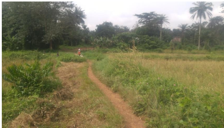
Figure 3.1: Vegetation on road; road reduced to a track
