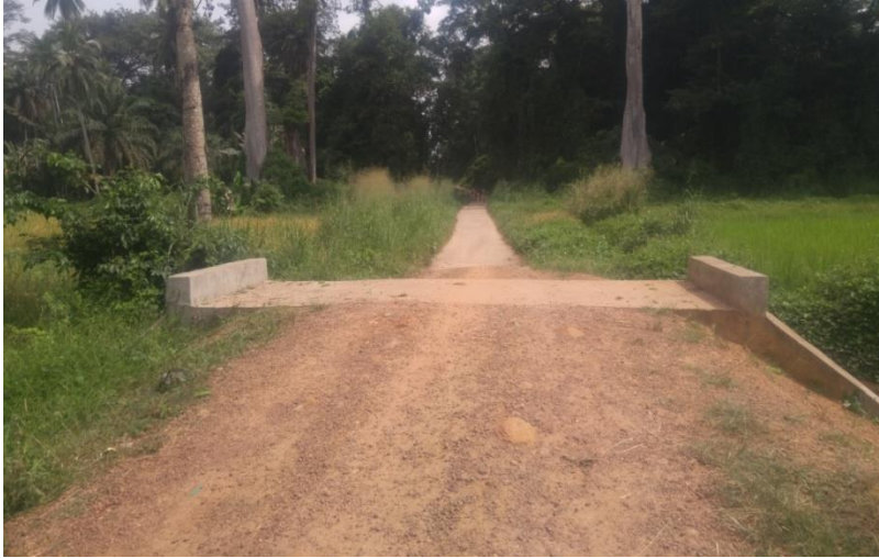
Figure 3.4 Road with Newly Constructed Culvert
